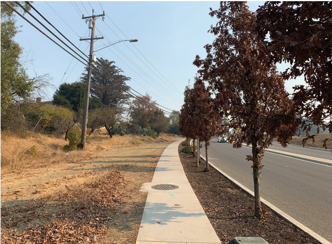
Photo 2: View of the project site from the west along Carlos Bee Boulevard.
