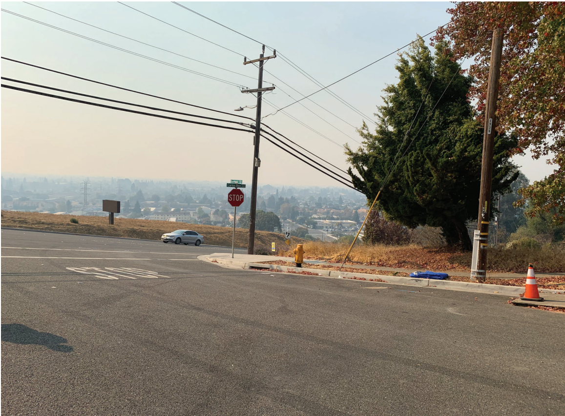
Photo 6: View of the Carlos Bee Boulevard and Overlook Avenue intersection from the east of the project site.
