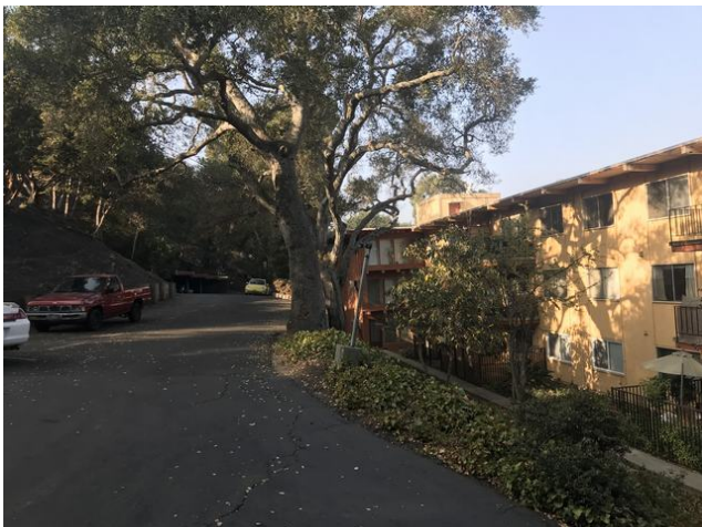
Exterior of Subject
