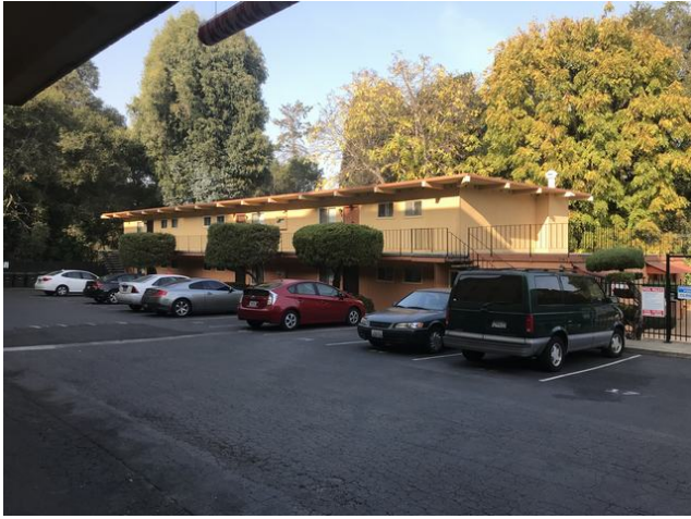
Exterior of Subject
