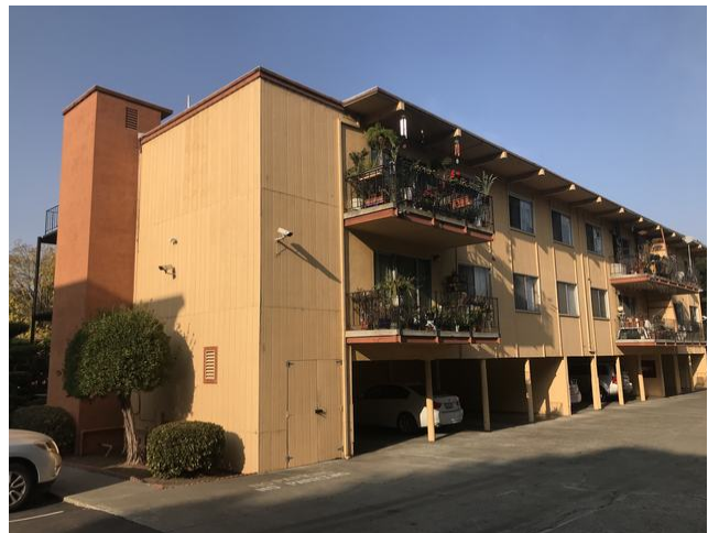
Exterior of Subject
