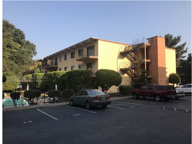
Exterior of Subject
