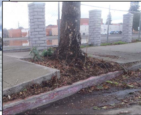
Photo 2 (L): Looking north at street trees #2-5 (background to foreground). These semi-mature to mature Chinese tallowes had performed well, remaining relatively small beneath the overhead utilities. However, all had displaced the surrounding sidewalk, curb and gutters from ~1" to 10". Inset shows base of street tree #2, which had lifted the sidewalk by ~8".
