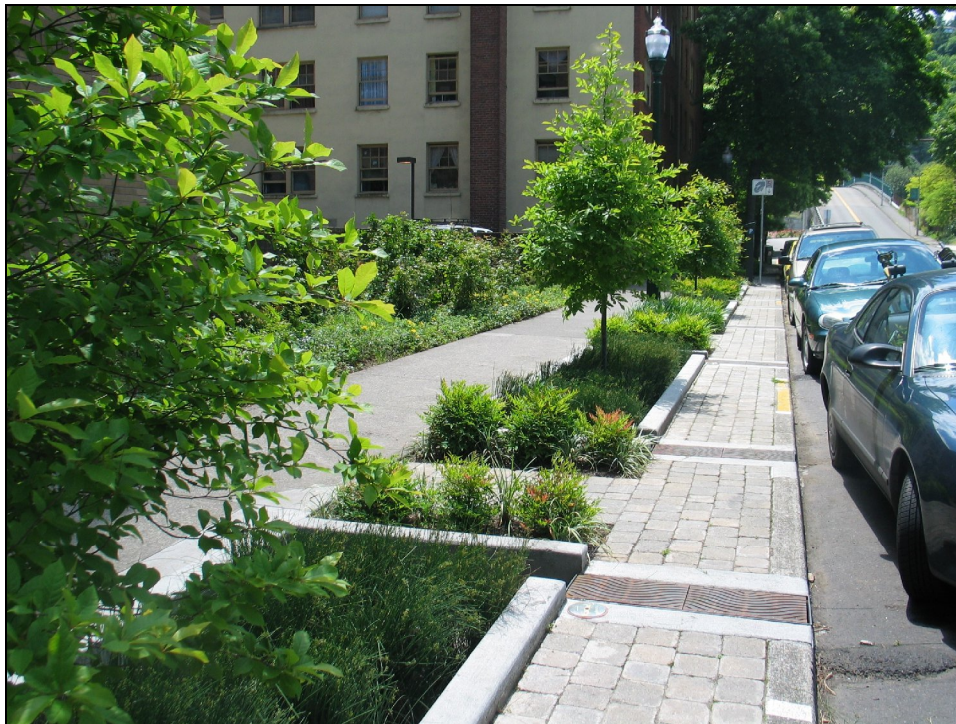
EXAMPLE OF BIOSWALE AND PERVIOUS PAVEMENT
