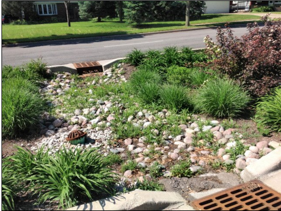
EXAMPLE OF BIORETENTION
