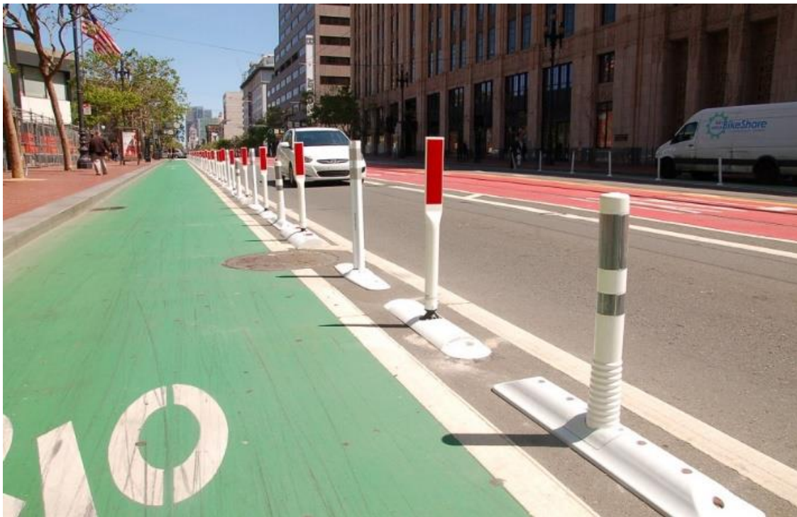
Figure B: Safe-hit delineator posts and painted bike lanes
