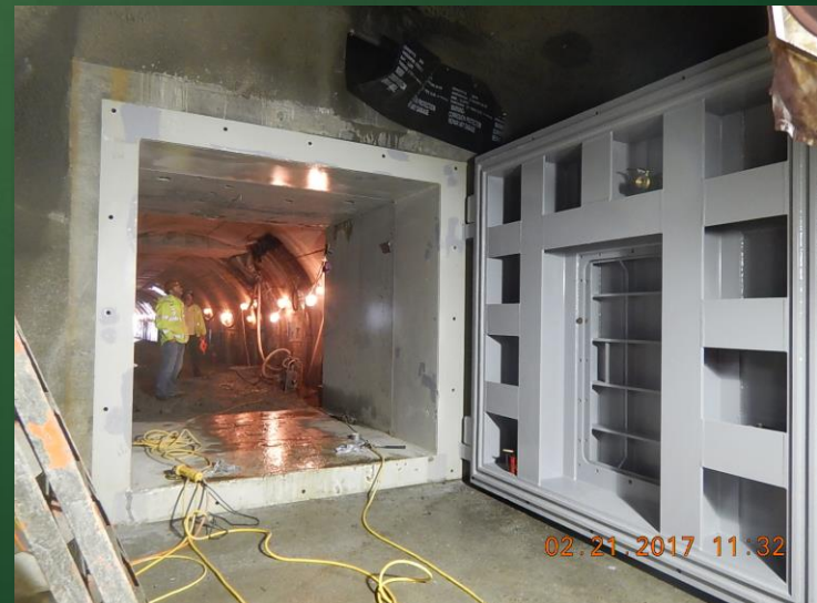
Completed New Adit Bulkhead
