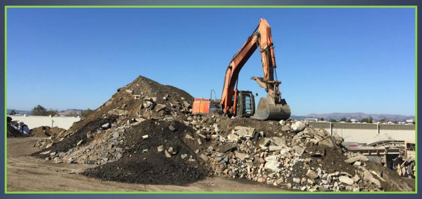
Excavator on top of stockpile. Noise Study prepared for the Depot Site recommends that use of the excavator should be at least 40 feet from the property line to be under 70 dba.
