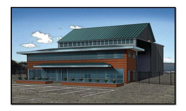
As part of this project, the former American Aircraft Sales office structure at 21015 Skywest Drive will be updated and modernized. Features will include expansive glass panels, stainless steel design details, and complete interior renovations. A new hangar will be constructed adjacent to the office structure that will accommodate a variety of aircraft.
