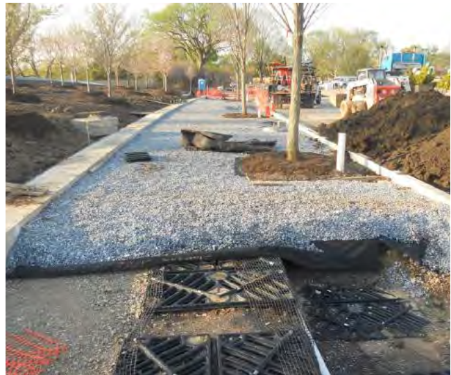
Silva Cell Installation ( http://www.deeproot.com/blog/blog-entries/sacred-memorial-20-years-in-the-making-silva-cell-case-study )
