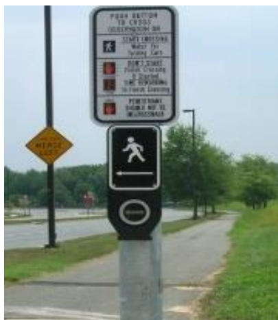
Accessible pedestrian signal push button with informational sign. Source: Montgomery County Department of General Services
