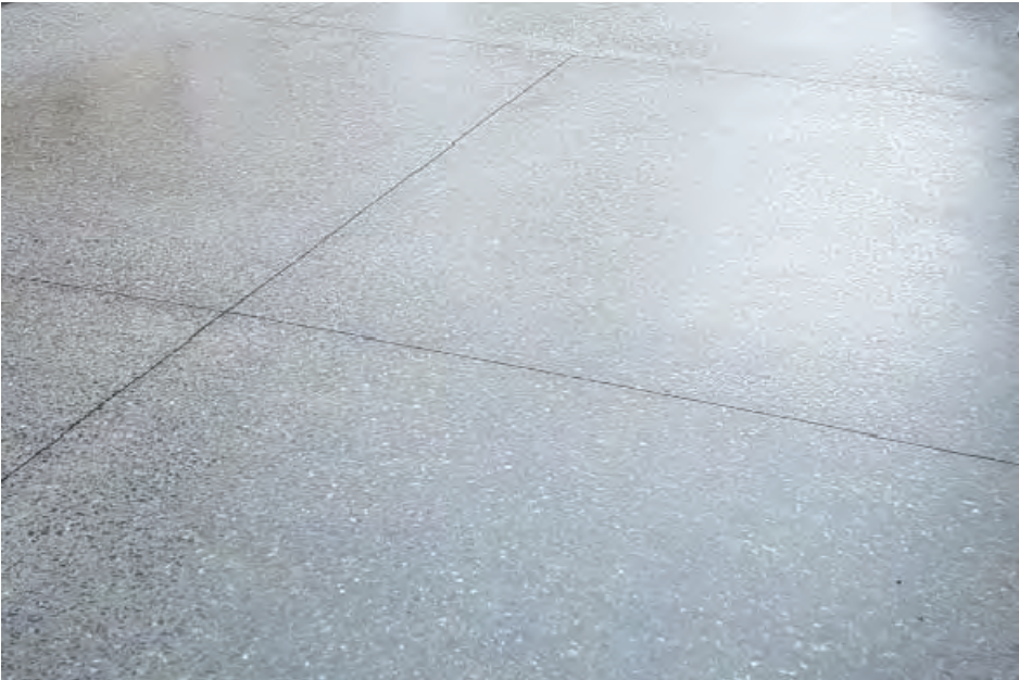
ACID-ETCHED CONCRETE PAVING
